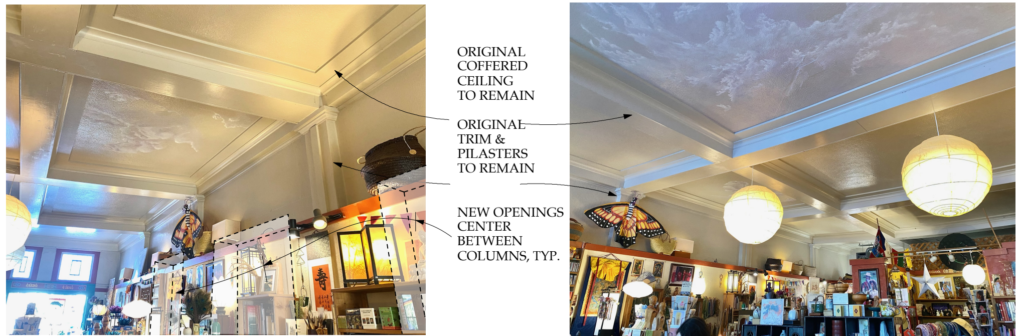
INTERIOR OF "OLD POST OFFICE" (735 8TH ST.) SHOWING COFFERED CEILING & PILASTERS
